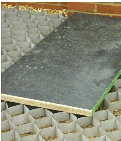
A timber board was placed on one grid, to ensure that it was in full contact with the ground before the aggregate fill was applied.
