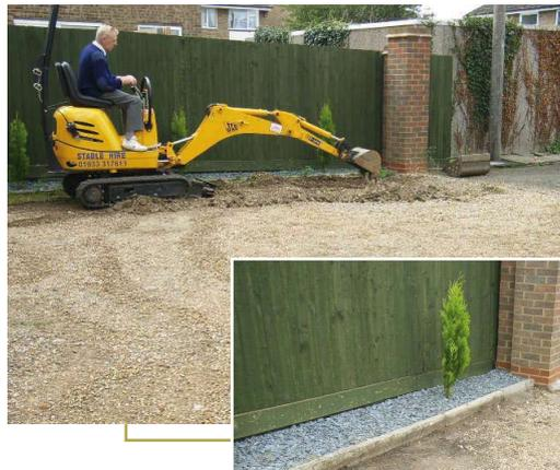
To relay the drive with DuPont™ Ground Grid, the ground was prepared first by removing approximately 65mm with a mechanical digger.
