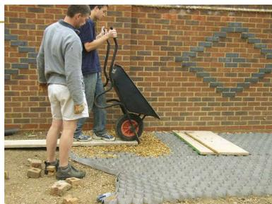
The aggregate was poured onto the grid manually, using a wheelbarrow, then raked in to fill the cells. The timber board was moved forward on the grid to continue the fill of the complete grid.
