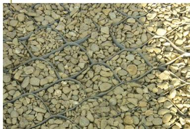
Once the grid cells had been filled to the top, the surface was stable enough to walk on to fill the rest of the grid, moving forward.
