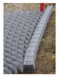
2) Next a Typar® geotextile was rolled out onto which GroundGrid® was then laid down. The geotextile prevents the filling material for the cells (crushed natural stones) from sinking down into the sandy subbase.
