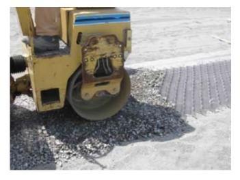
The stone layer was compacted one more time to ensure the cells were completely filled.
