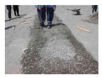
4) The last installation step involved covering the grids with a top layer of sand so that the access way integrates smoothly into the beach panorama.
